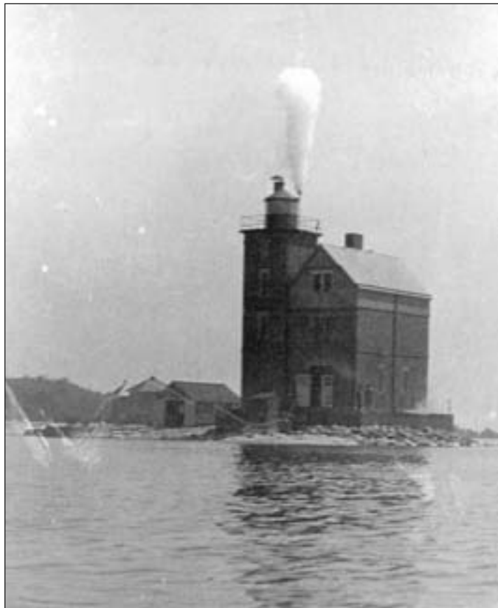
Steam used in the fog horn system rises from Round Island Lighthouse. (Photograph courtesy of Tom Pfeiffelmann)
