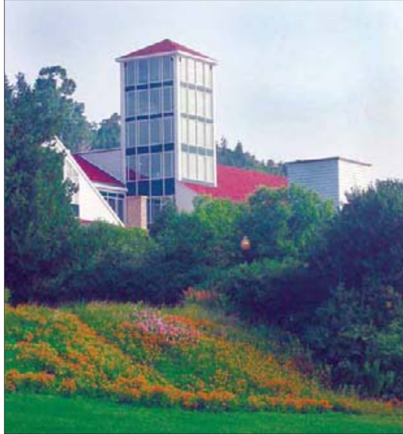
Mission Point's observation tower, which has long been a focal point of the resort, now features a new maritime museum exhibit.
