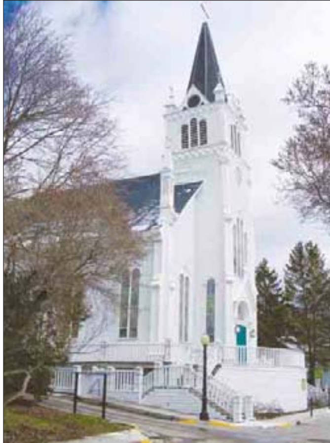
Money is being sought to renovate the steeple of Ste. Anne's Catholic Church, which rises 120 feet above Main Street. The building was constructed in 1874 and serves more than 70 registered Mackinac Island parishioners year-around. During the summer months, visitors are drawn to services at the parish, which is more than 300 years old.
