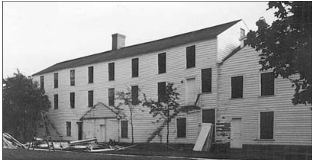
Mission House was one of the buildings Rev. Humbard purchased.
