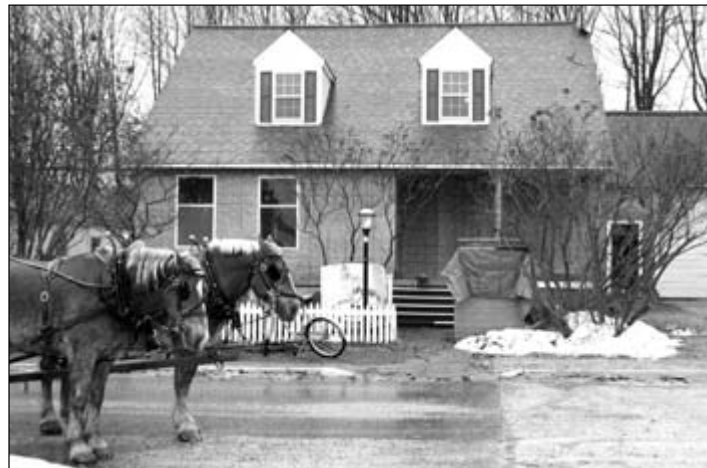
In preparation for new siding, plywood covers Mackinac Island's old medical center on Market Street. The building is being converted to housing for Island police. The fiber cement siding planned for the historic district structure raised concerns of city planners Tuesday, January 8.
